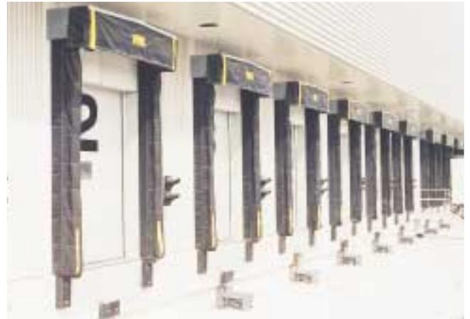
*Pentalift PSI-350 inflatable dock seals are durable and provide an effective seal.*
