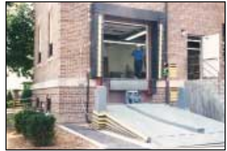
Surface Mounted Truck Leveler in the raised position.
